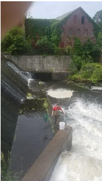
Seasonal Zack Skelton monitors the drawdown of the Somersville Dam Pond.
